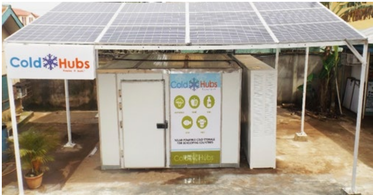
A solar-powered cold room prototype at Owerri Relief Market, Imo State, Nigeria. Photo courtesy of ColdHubs/Ikegwuonu.
