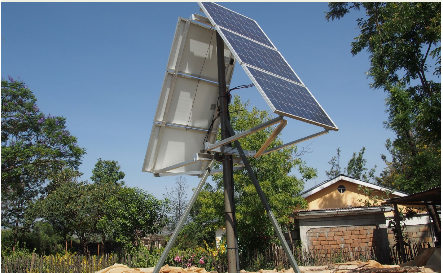
Powering Agriculture innovator SunDanzer's East-West facing panels create a flatter PV curve. Photo courtesy of SunDanzer.
