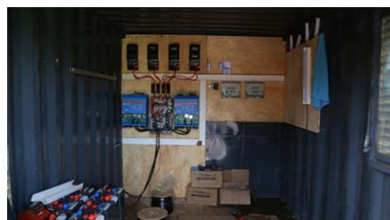
Kyamugarura mini-grid plant room during construction
